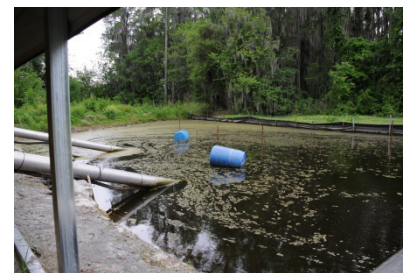
Figure 2. Inlet pipes run from irrigation ponds. Note the blue barrels that are keeping the ends of the pipe from sitting on the bottom of the pond.
