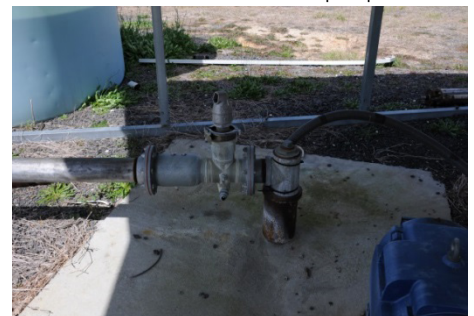
Figure 3. The wellhead should be inspected prior to a freezing event.
